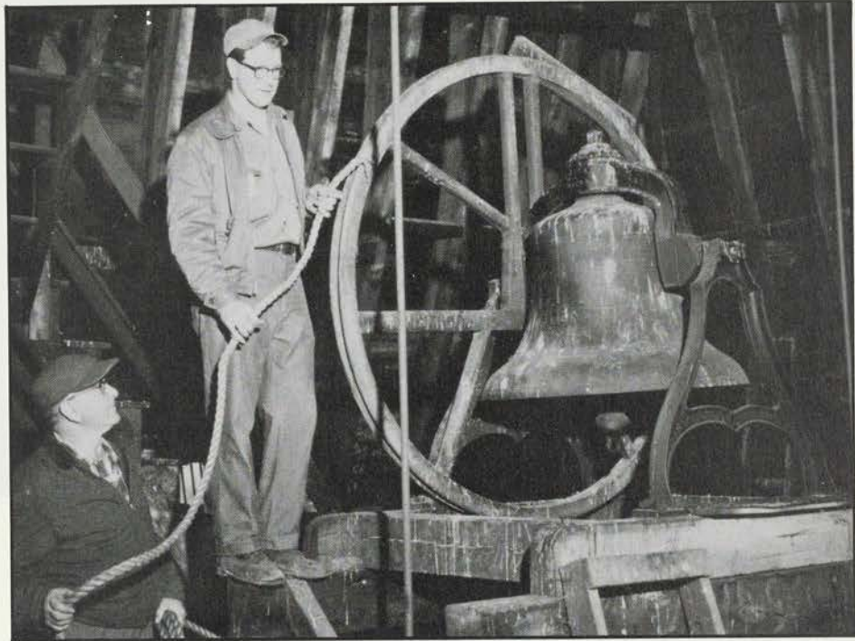
The campus bell hung in the tower of Old Main where it was rung with a rope on a wheel. Henry Herr, the younger man above, still works on the university grounds crew and loaned the Review several of the photos in this article.
